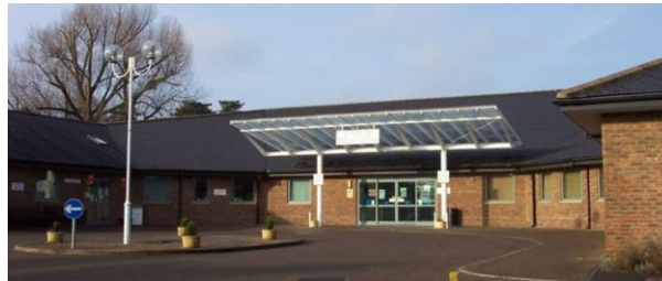
Chepstow Community Hospital opened in 2000 having been developed under the Government's Private Finance Initiative.
